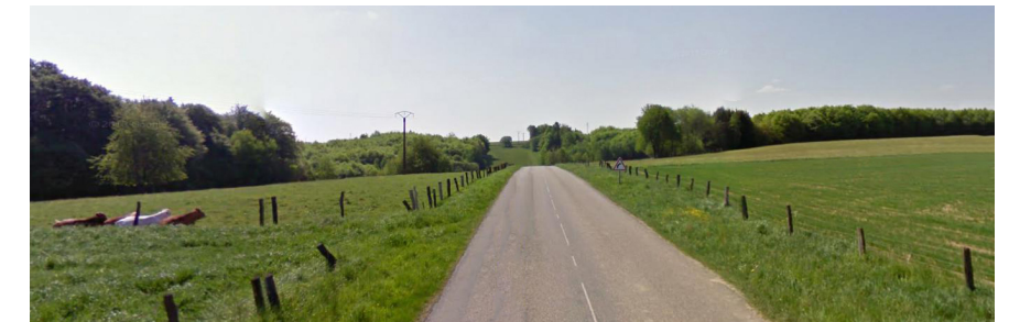
Photo 82: 1 – Amont Grandrupt RD164 - direction Gruey (Source : Google Earth 2011)
